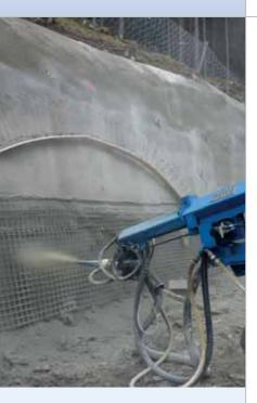
Set/hardening accelerators and set accelerators for sprayed concrete must correspond to the common requirements set out in EN 934-1 and the specific requirements in EN 934-2 or EN 934-5. They are defined here as:
